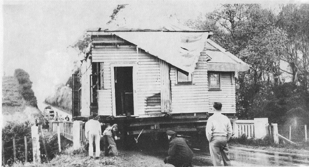
A section of the house owned by Mr F. Butler being moved from its Gill Street site to a new site on Mountain Road. It looked a tight squeeze when a small bridge across the Mangaoraka Stream, just north of the New Plymouth airport was reached, but the solution proved simple and the tray of the transporter was raised a couple of inches. Traffic Officer Ross was kept busy guiding traffic and all was well in little over an hour when Mr Wallis, a Hawera Contractor was able to breathe again as the first section of the house was delivered to its new home. The other half was moved later proving that in these days one can always pick up ones house and find fresh pastures.
