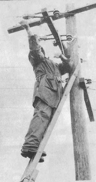
Removing fuses from power lines lifting wires with bamboo pole.
